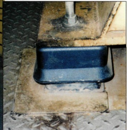
Figure 16 Detail of anti-vibration mount
